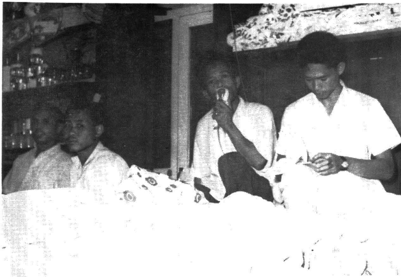
Shoping Centre Pasar Senen (1967)
