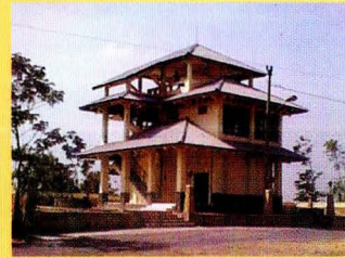
Fig. .64. Facility construction
