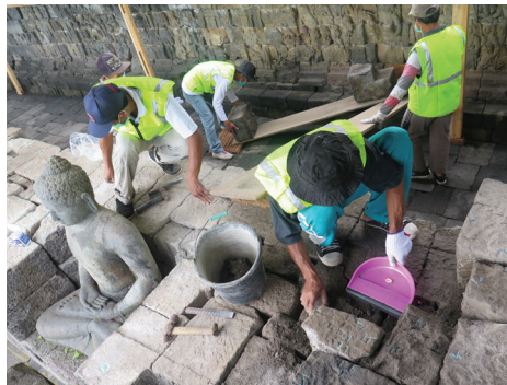
Penanganan kebocoran Candi Borobudur
