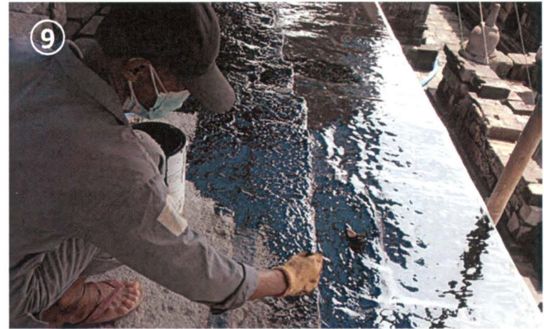
Photo 9. Applying Araldite Tar on the lead plate and stone.
