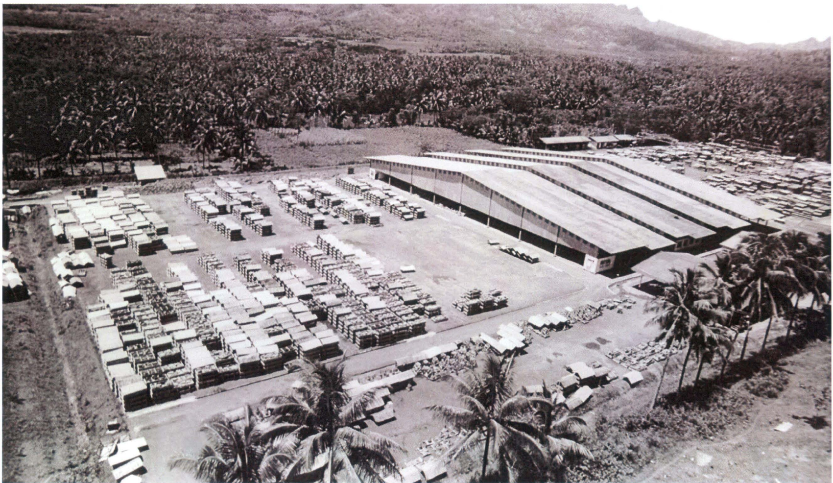
Area buffer storage, workshop dan final storage (dari kiri ke kanan).
