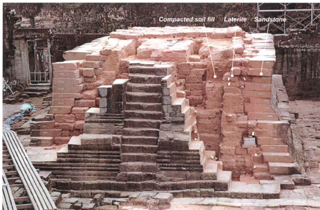
Photo 12. After partial dismantling of the upper structure and corners of platform, Southern Library of Bayon, restoration by JASA in 2006-2011
