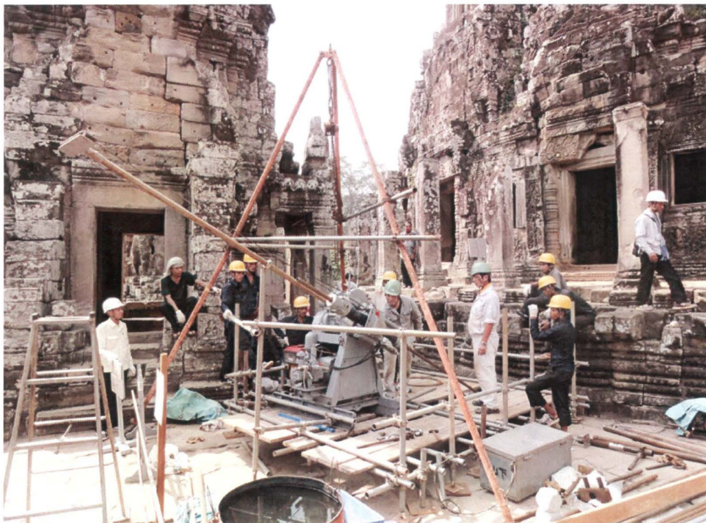
Photo 13. Boring survey at the Central Terrace of Bayon by JASA (2011)
