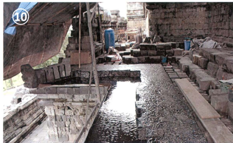
Photo 10. Water leaking test under balustrade.
